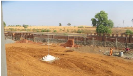
Construction of the compound wall
